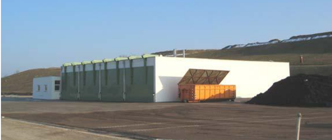
Biogas plant, dry fermentation type, batch system.
