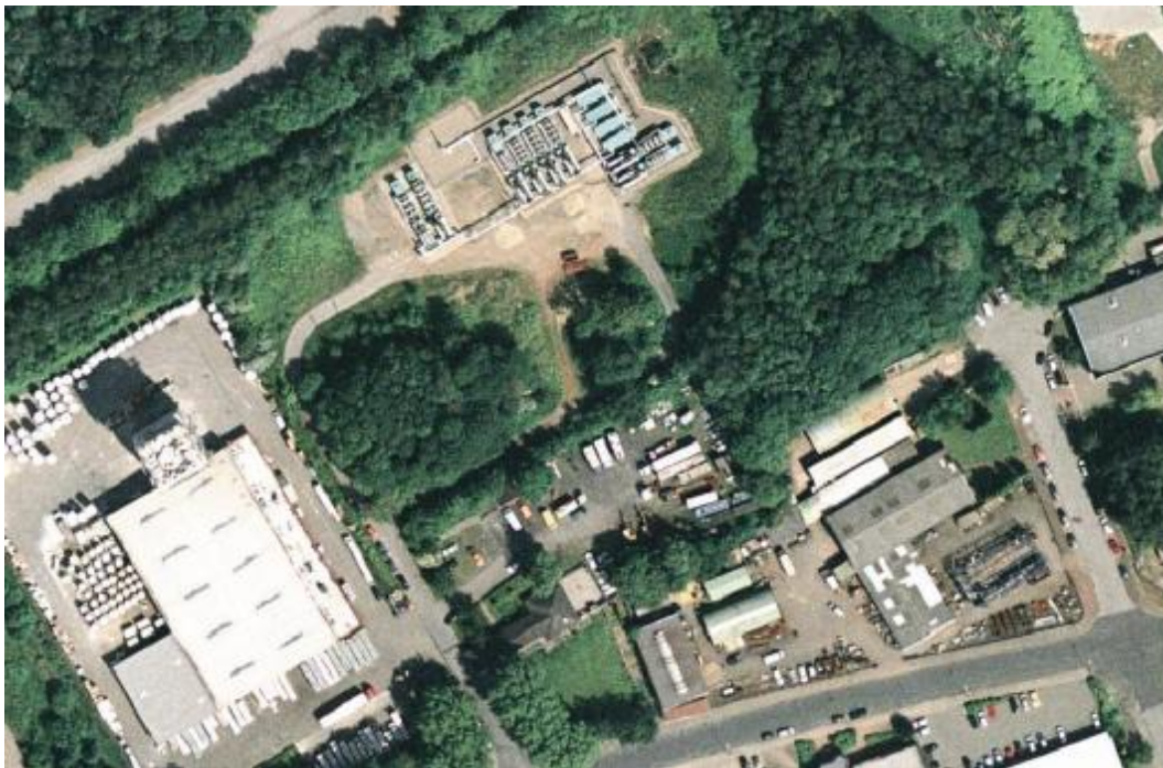
Mine gas plant nearby buildings.
